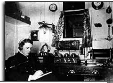
An unidentified wireless operator in a shipboard Marconi telegraph room probably similar to the Titanic 's. By 1912, all North Atlantic passenger ships carried wireless equipment.
